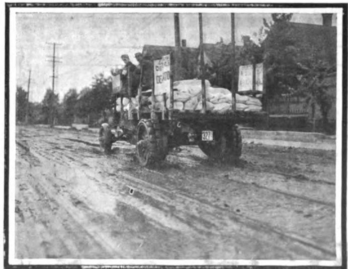
The heavy trucks weathered the mushy streets without great difficulty
